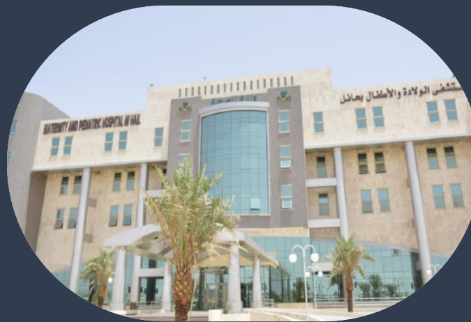
Hail Maternity Hospital Project
